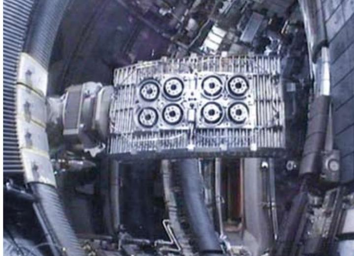
Fig. 1 The ITER like antenna during installation in JET
